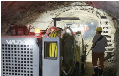
陕西潼鑫矿业金矿 断面: 2.6m×2.6m
